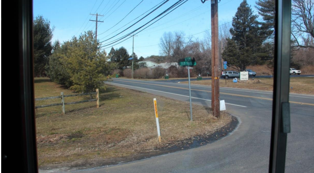
Figure 16. School bus driver sight distance (206 feet) from white stop line on northbound BCR 660.
