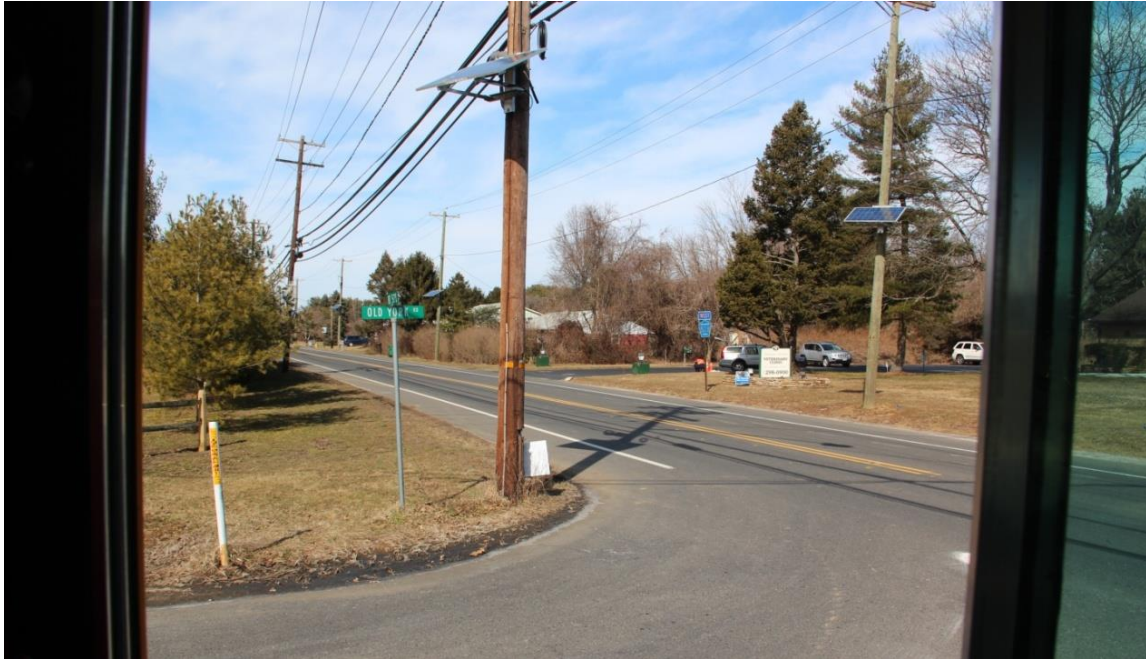
Figure 17. Sight distance from likely school bus driver stopping position on northbound BCR 660.
